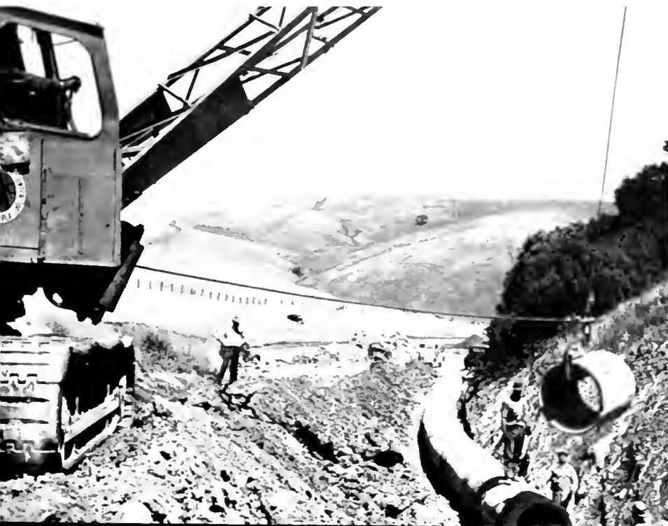
Dragline placing 36-inch reinforced concrete drainage pipe
